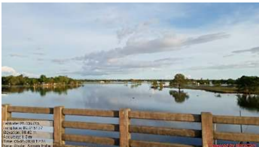
Figure 6: image of existing major bridge at chainage 51+536km
